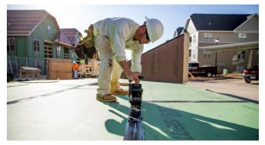
Installers pre-assembled ZIP System<sup>®</sup> sheathing panels and tape before installing on exterior walls and roofs.
