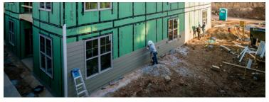
With a built-in water resistive barrier, ZIP System<sup>®</sup> sheathing and tape saves installation time by eliminating housewrap.
