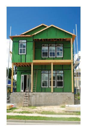
ZIP System sheathing and tape is an innovative structural roof and wall system with an integrated water- resistive barrier that streamlines the weatherization process. The system helps Sapphire Homes get projects dried in quicker in the rain-heavy Gulf Coast area.
