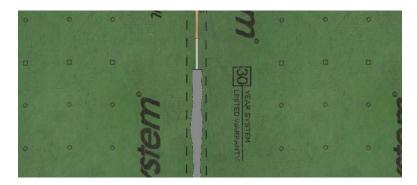
\*Pro Tip: when using ZIP System liquid flash, install a bead into the groove over the backer rod and then apply a bead on either side of the joint to ensure proper mil thickness and width of ZIP System liquid flash.
