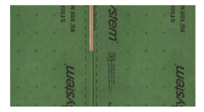
Step 2: Install the ZIP System flashing tape or ZIP System liquid flash over the filler stip. Ensuring a minimum of 1-inch of coverage is achieved on to the ZIP System sheathing or ZIP System R-sheathing panels on either side of the joint.
