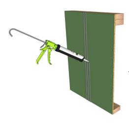
Once applied into the joint, place a bead of ZIP System<sup>™</sup> liquid flash approximately ½" away from the joint on either side of the seam. This can be done in a straight line or in a serpentine pattern.
