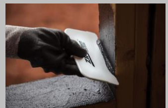
ZIP System™ liquid flash is fluid-applied flashing that flows into hard-to-flash areas for an air- and water-tight seal.
