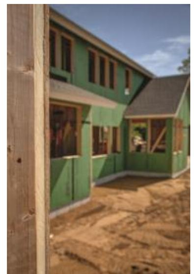
was quickly adopted by progressive, energy-efficient builders across the country who have been able to prove the significant contributions ZIP System R-sheathing and tape has made to help provide higher R-value and reduce air leakage. Massachusetts Passive House architect Steve Baczek has used ZIP System R-sheathing in multiple high-performance, net-zero homes.
