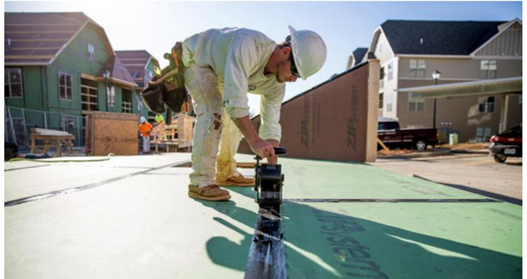
*Installers pre-assembled ZIP System® sheathing panels and tape before installing on exterior walls and roofs.*
